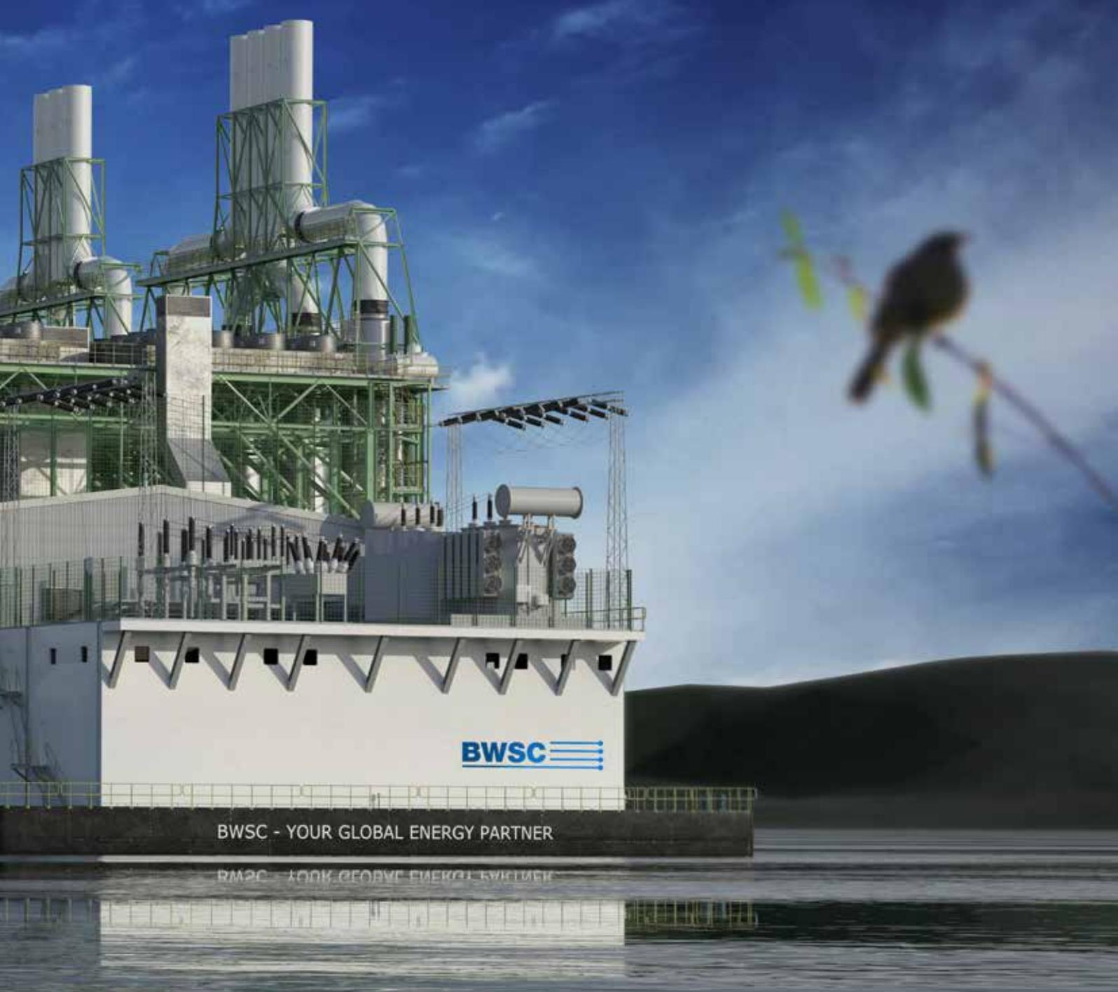
The power barge will supply the FSRU with electricity and hot water for re-gasification.
