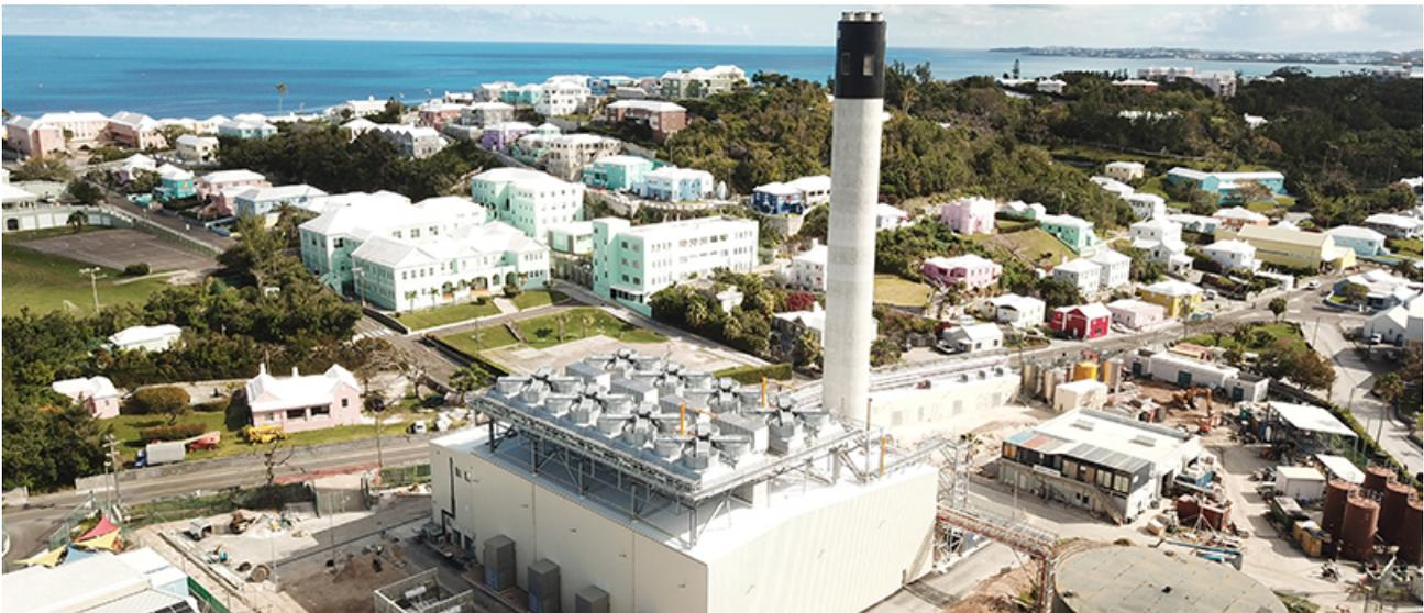
BWSC has a history with BELCO going back to the first contract in 1982. Since then we have had several contracts with BELCO, including East Power Station with 2 x 12.8 MW low speed engines in 1984 and 1985, 2 x 14.8 MW in 2000 and 2 x 14.8 MW in 2005. Further, we have had several service activities at the Pembroke Power Station site, including a 5-year service agreement with spare parts, upgrade and maintenance works – latest the ongoing repair of two of the East Power Station radiators.
