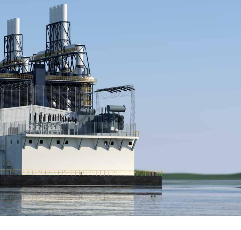
The power barge will supply the FSRU with electricity and hot water for regasification.
