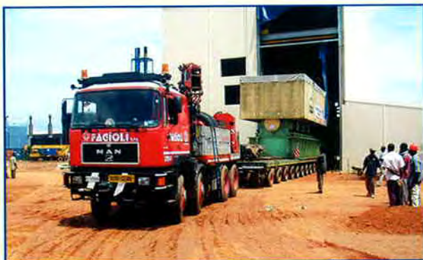
Offloading engine at site
