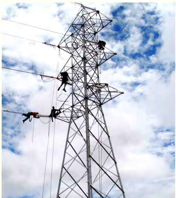
Men working on transmission lines
