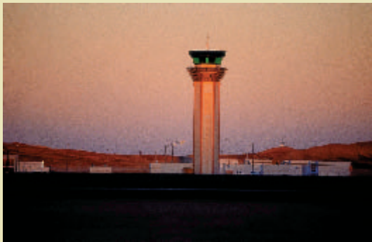
New Marsa Alam International Airport.
