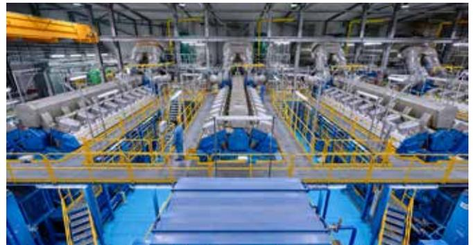
Four Wärtsilä 18V46 high-performance, medium-speed, 4-stroke HFO diesel engines
