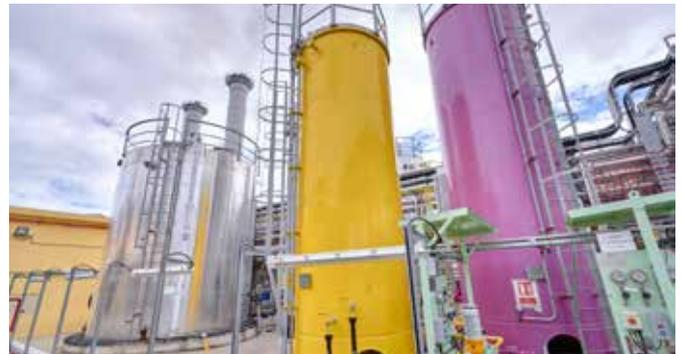
*Service tank farm – diesel oil, heavy fuel oil, lubricating oil and sludge*
