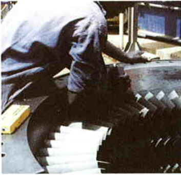
▲ Modification of the turbine stator during pre-test of the power plant.
