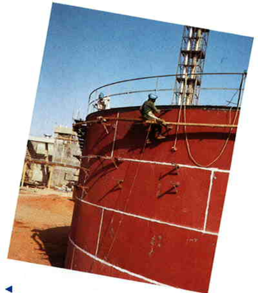
◀ Erection of radiator cooler, air intake filter and exhaust stack for turbine.
