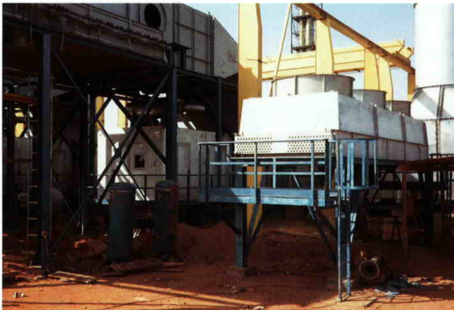
◀ Erection of radiator cooler, air intake filter and exhaust stack for turbine.
