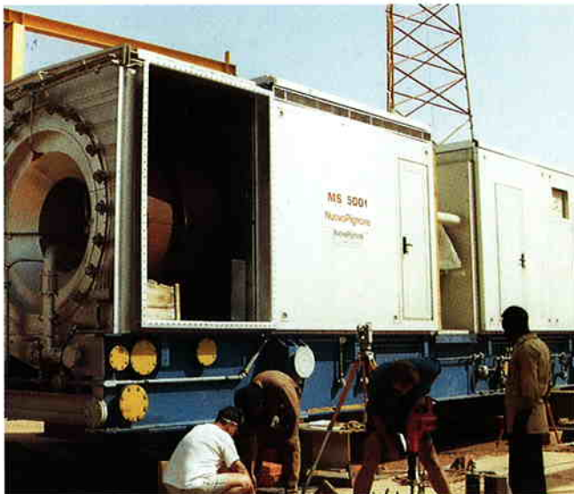
▲ Preparation of foundation before installation ► of gas turbines and generators
