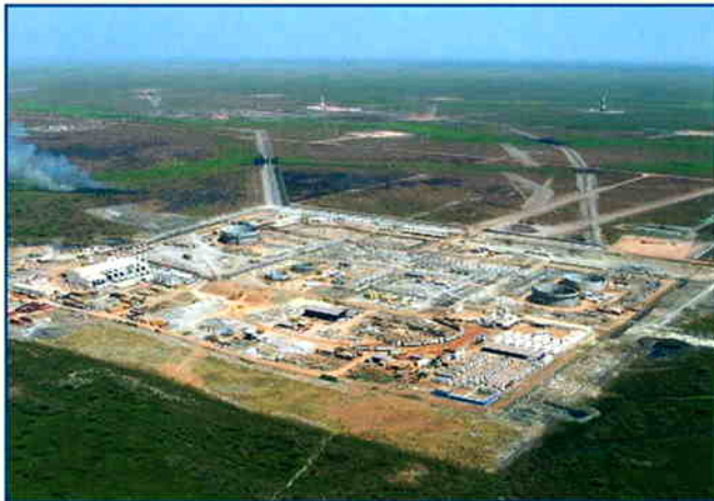
WNPOC Crude Oil Treatment Plant Under Construction
