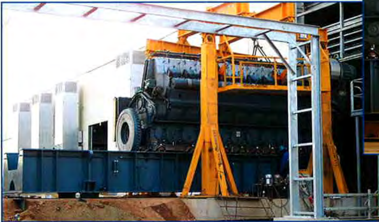
Ganty crane in operation
