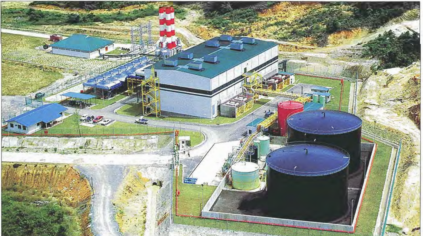
Aerial view of the entire Plant
