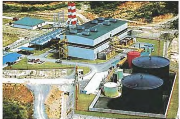
Libaran Power Station (Malaysia)
