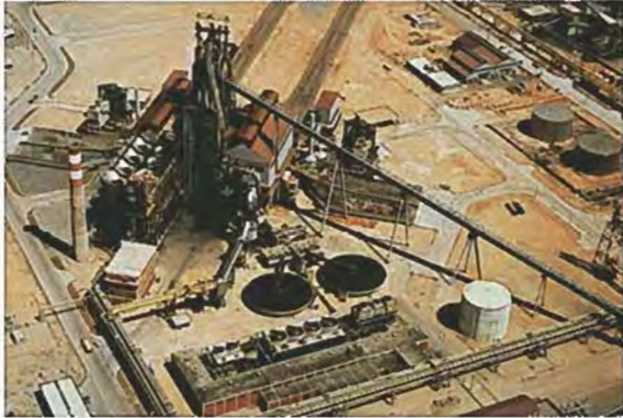
Tubaron Steel Mill (Brazil)
