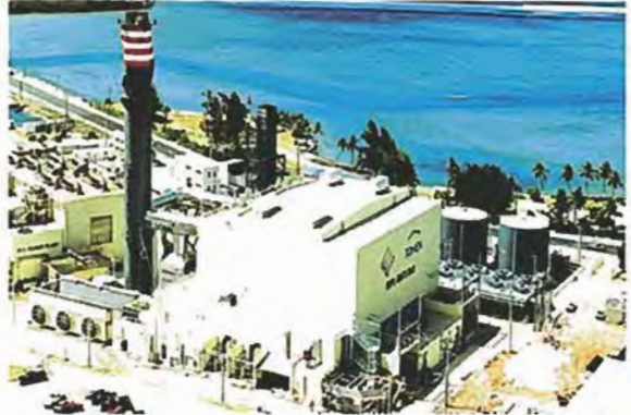
Guam Piti Power Station
