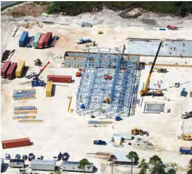
Modularization concepts were utilized for design, manufacture, logistics and construction in order to complete the plant within the contractual time frame of 13 months for the first three generating units and 14.5 months for the remaining three generation units.
