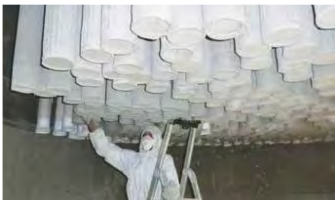
Inside FGD bag-house filter.
