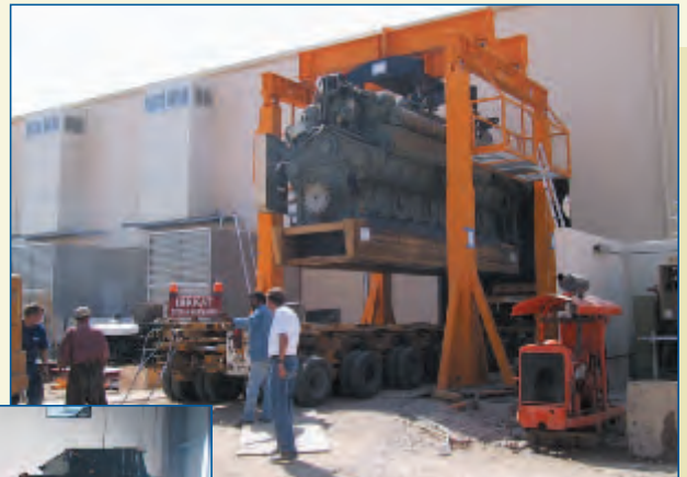
Engine unloading at site
