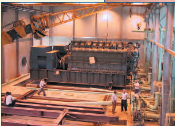
Engine on foundation
