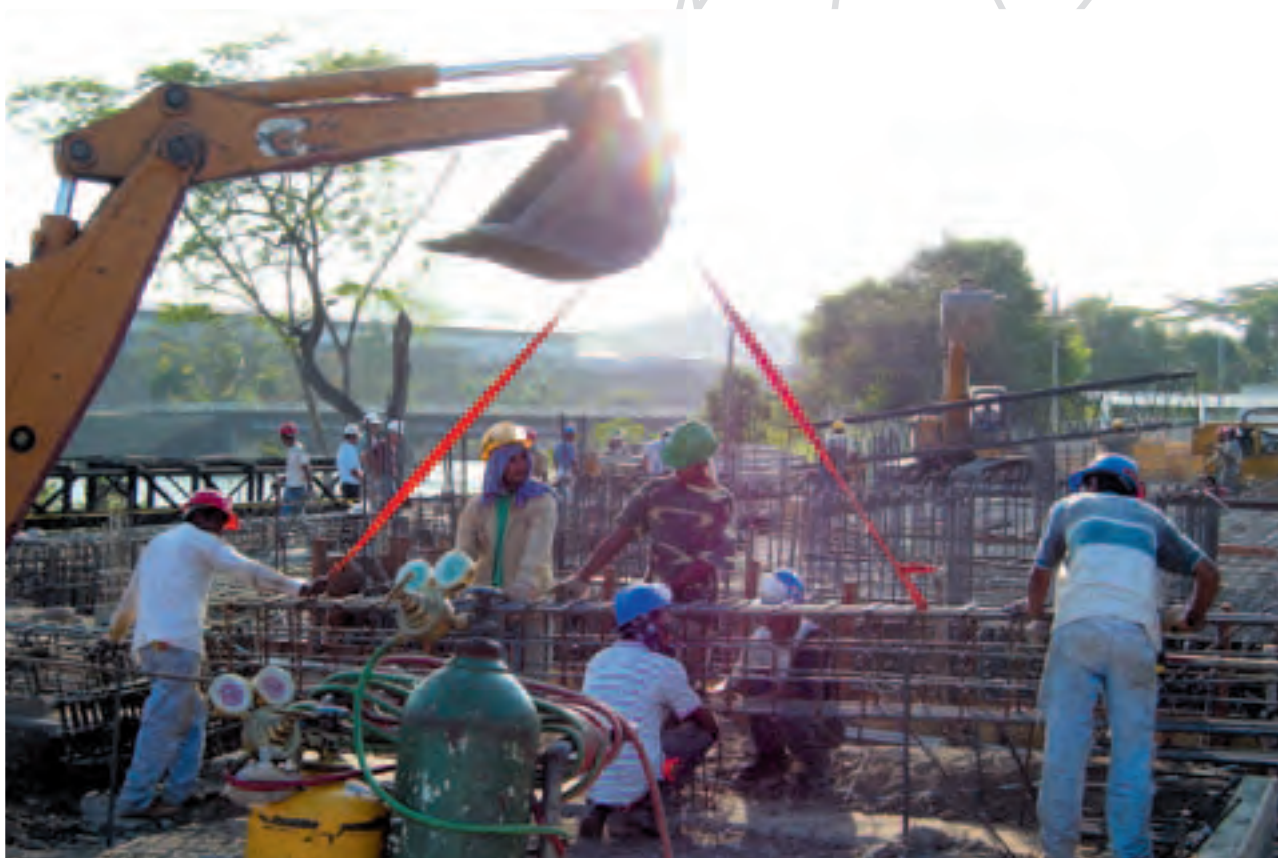
Miraflores Power Station in Panama under construction.
