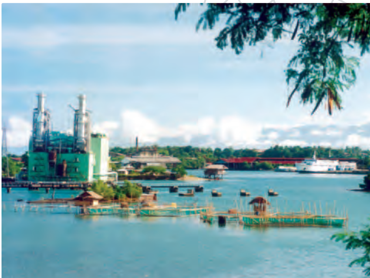
Mindanao Power Barge, the Philippines.
