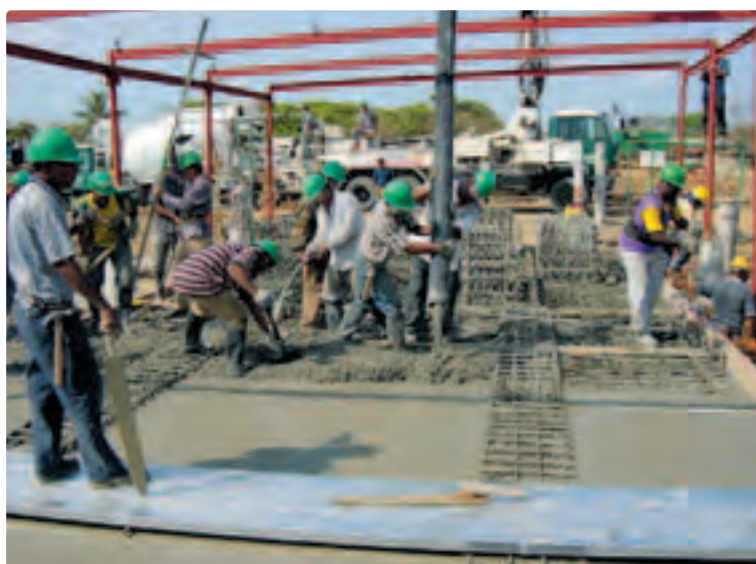
Pacora Power Station in Panama under construction.
