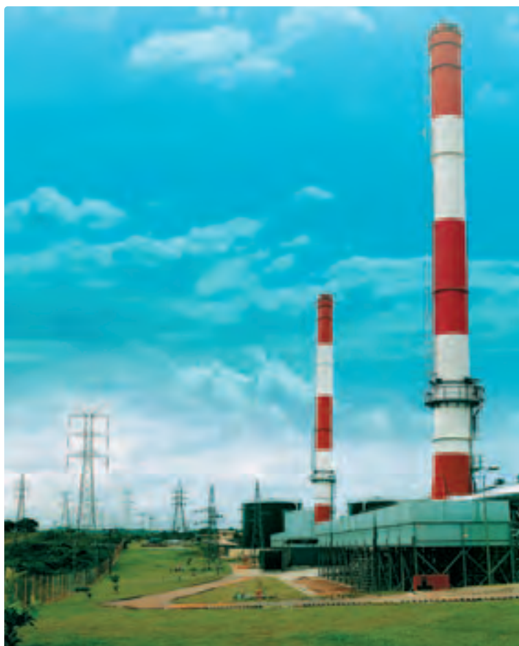
Sapugaskanda BOO Power Station in Sri Lanka.
