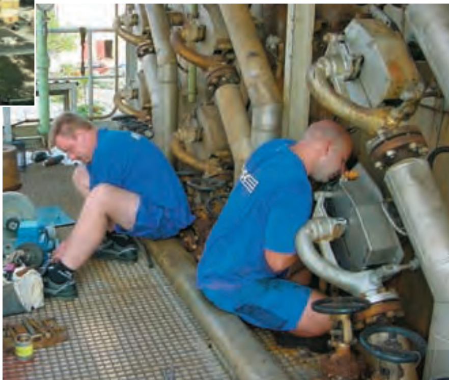
Clifton Pier Power Station, the Bahamas - overhaul of soot blower.
