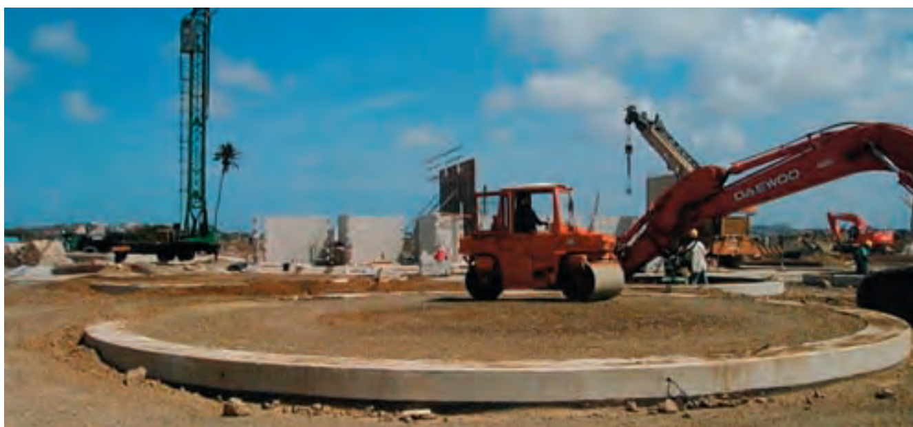
Tank Foundation, Curacao Power Plant under construction.
