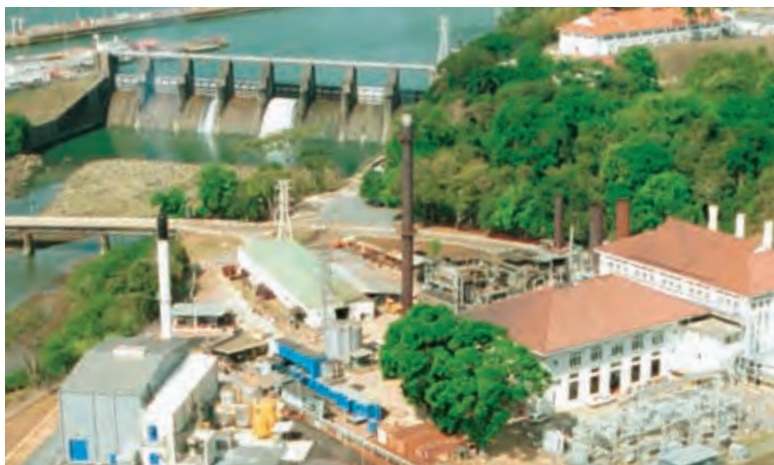
Miraflores Power Station, Panama.
