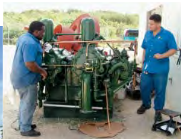
Renovation of Carribean Utilities Co. LTD. 's first diesel engine on Grand Cayman to be used for exhibition purposes.
