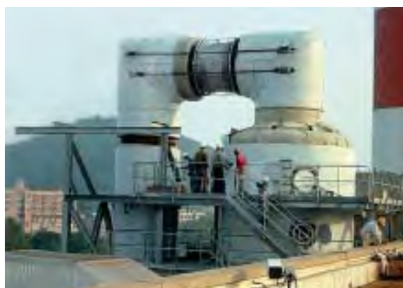
Selective Catalytic Reduction System (SCR) for Coloane Power Station, Macau.
