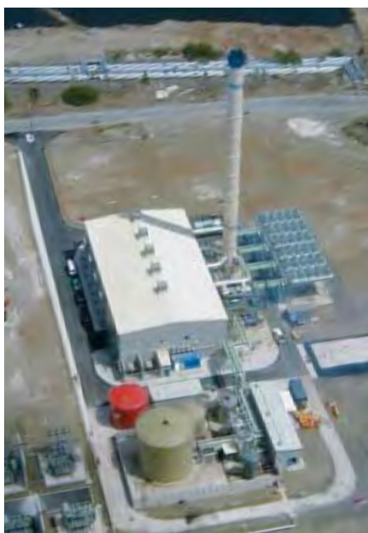
Aqualectra Diesel Power Station, Curacao.
