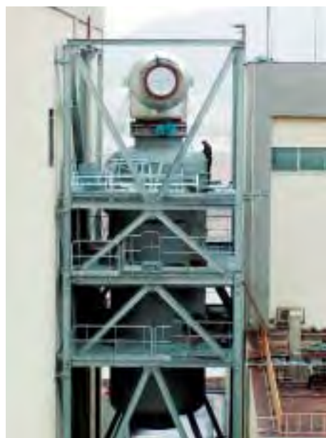
SCR reactor under installation.
