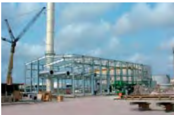
Powerhouse structure, Curacao.
