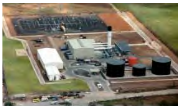
Aerial view of Pacora Power Station, Panama.
