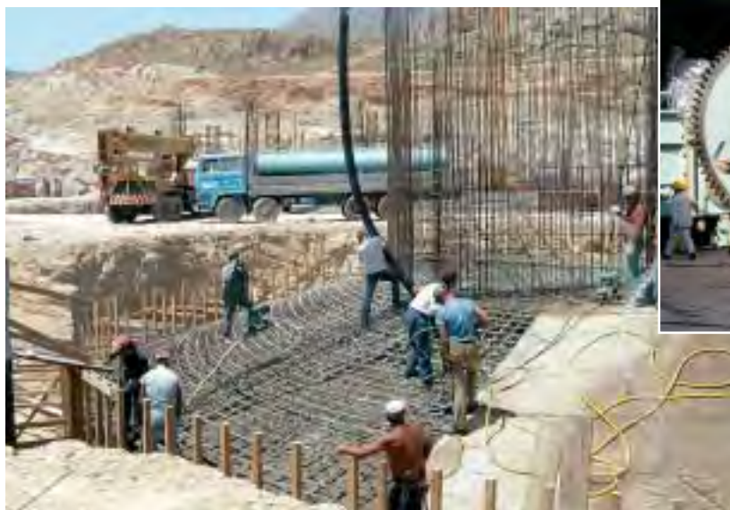
Atherinolakkos 102 MW Diesel Power Station under construction, Crete, Greece.
