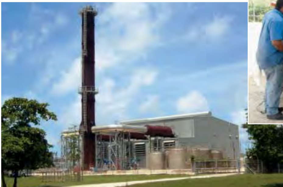
The North Sound Road Power Station, Grand Cayman Island.
