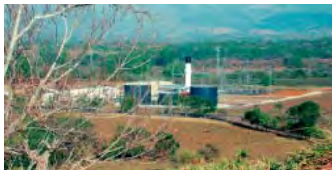
The site of Pacora Power Station.
