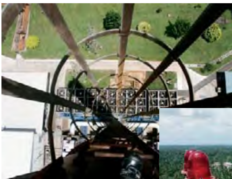
View down from top of stack, Asia Power Station, Sri Lanka.
