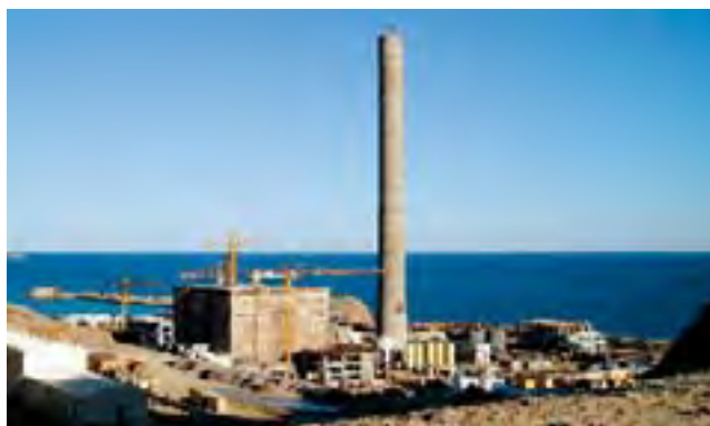
Atherinolakkos Power Station under construction, Crete, Greece, January 2004.
