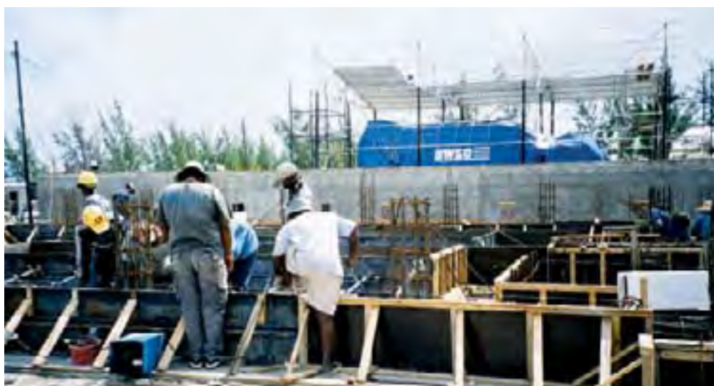
Pointe Monnier Power Station under construction, Rodrigues, Mauritius.
