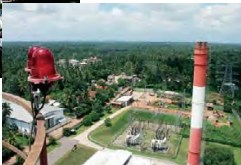
View from top of stack, Asia Power Station, Sri Lanka.
