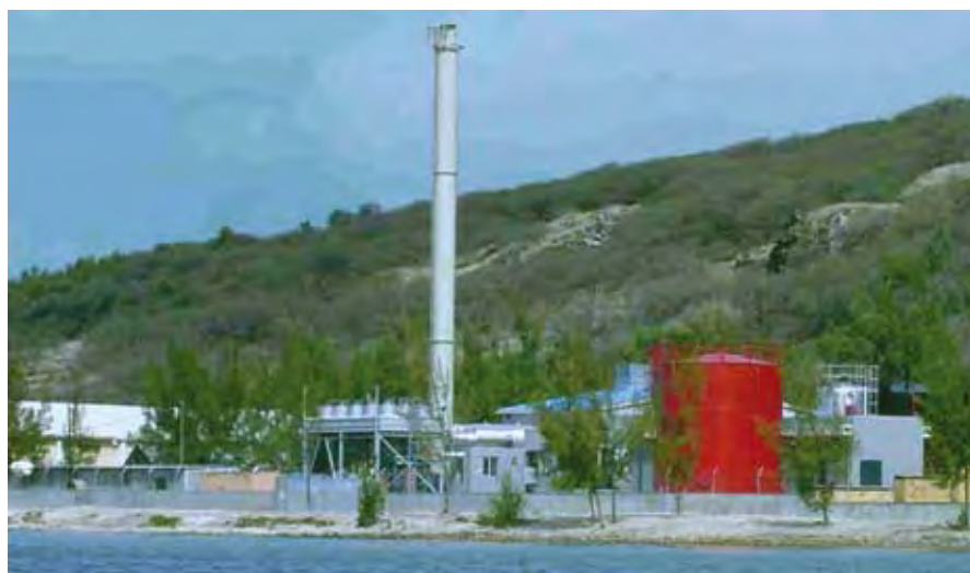
Pointe Monnier Power Station, Mauritius
